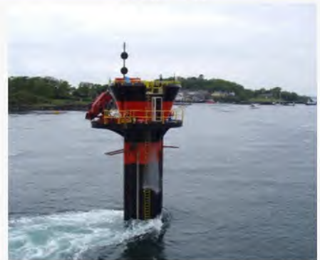
Commercial tidal stream generator — SeaGen — in Strangford Lough . The strong wake shows the power in the tidal current.
